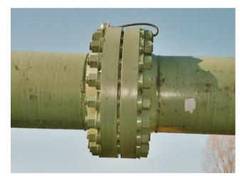
The inspection is impossible for the pipe including a flange and valve in penetrated section.
